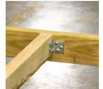
**TIP:** Attach the brackets in the center of the 2x4s for maximum strength
